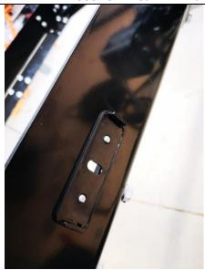
The wires get fed through the hole in the bracket and then the light snaps into place onto the bracket
