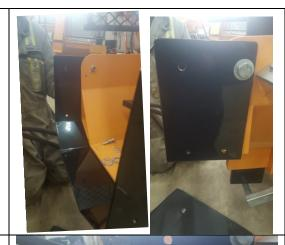
Install upper winch bracket, line up lower holes and install bolts
